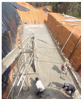
The foundations and floor of another massive underground water tank to catch all the rain water which is used for drinking in the various houses around that area. This will be our 14 th underground water tank.
