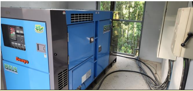
One of our two new generators which generate 125 KVA. These incredible machines are a wonderful gift from a few people around the world.
